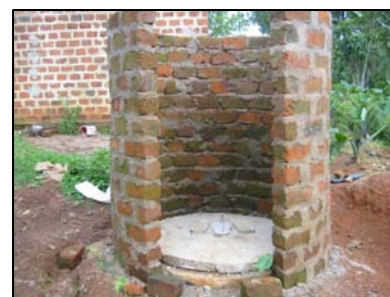
Figure 9.5: URCD toilet with super structure at RASD
