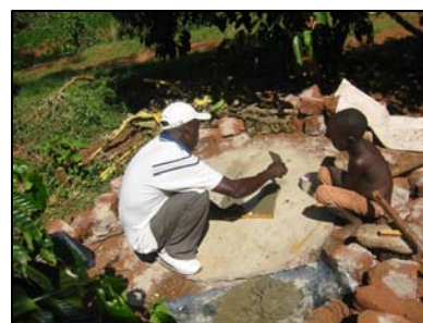
Figure 9.9: The construction of URCD toilet near RASD
