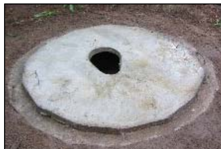
Figure 9.3: Squat plate for pit latrine Source: Morgan, 2007
