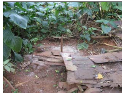
Figure 7.1: Pit latrine with a makeshift wooden slab
